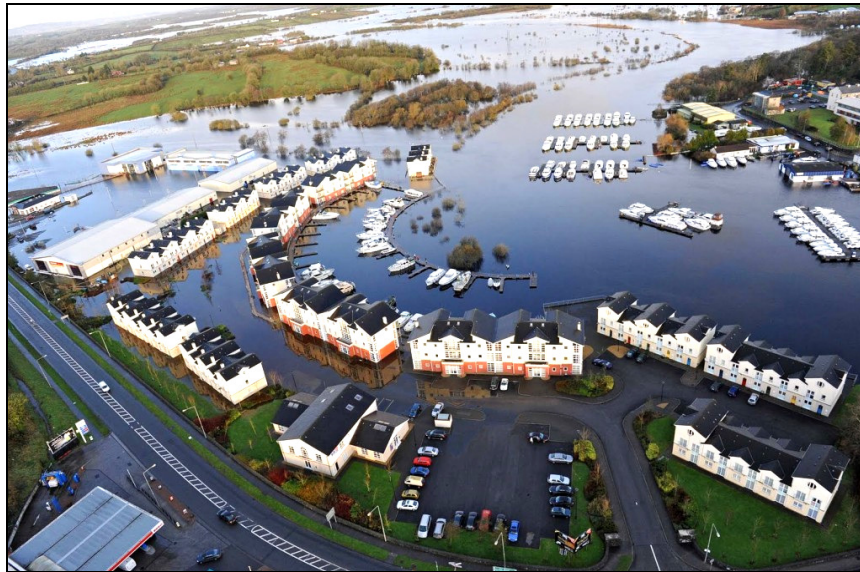
2009 - Severe Flooding in the West of Ireland
